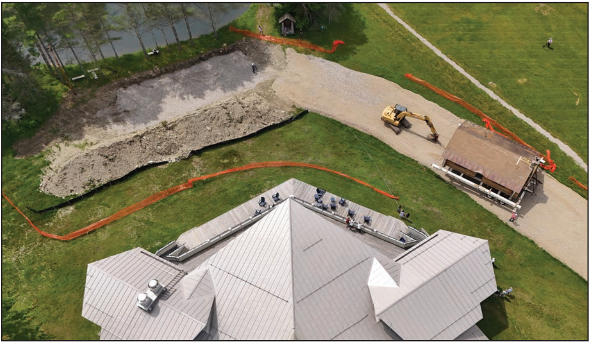
THIS BIRD’S-EYE VIEW at the Snowbowl shows the Hubbard Cabin as it is pulled to its new location near the snowmaking pond (top left) in front of Starr Lodge.
