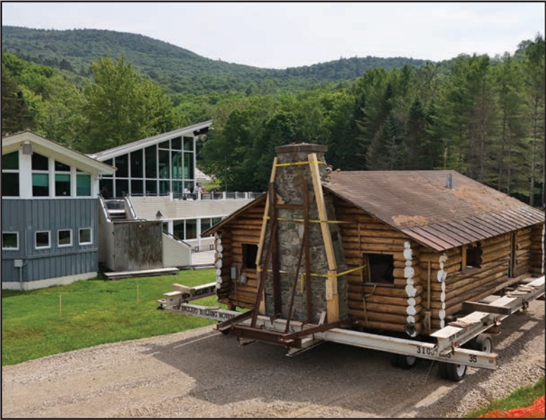
NEW ENGLAND BUILDING Movers, with help from M. Gale Buildings, put the Hubbard Cabin on steel beams, planks and wheels so it could relocate the structure.
