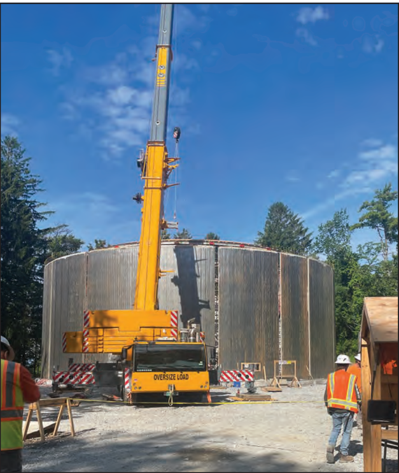
WORKERS FROM DN Tanks LLC are using a massive crane to hoist large concrete panels to form the dome of the new 1.3-million-gallon municipal water tower that’s being completed on Chipman Hill in Middlebury.
