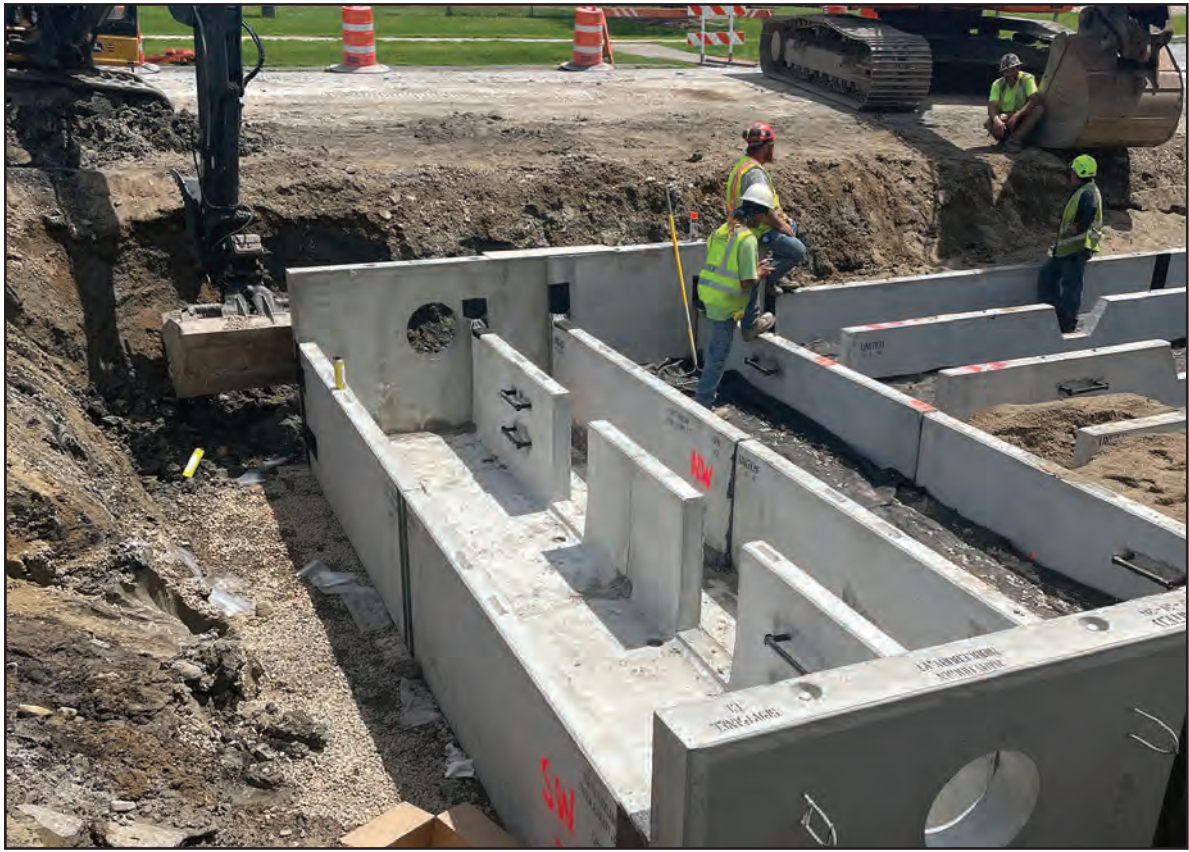
HERE WE SEE workers complete a segment of a new stormwater treatment system that will process runoff from four acres of impervious surfaces on the Mary Hogan Elementary School/recreation park property in Middlebury.
