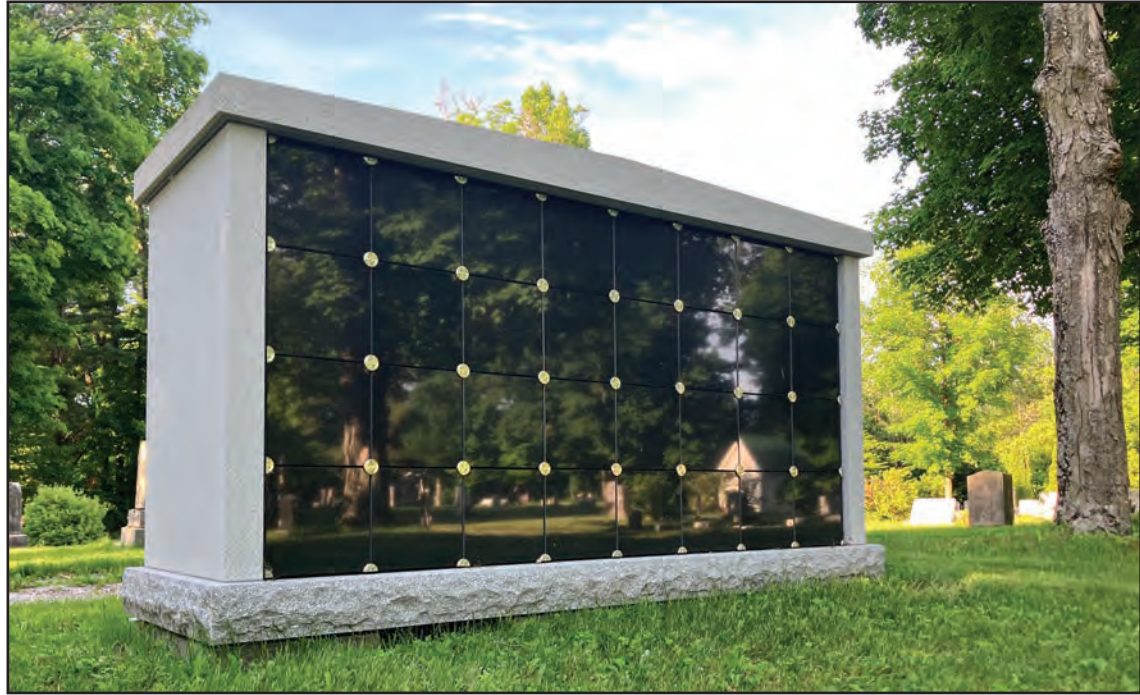
GRAY AND BLACK granite in a new columbarium at Prospect Cemetery in East Middlebury houses 64 niches where families can store the ashes of cremated loved ones.
