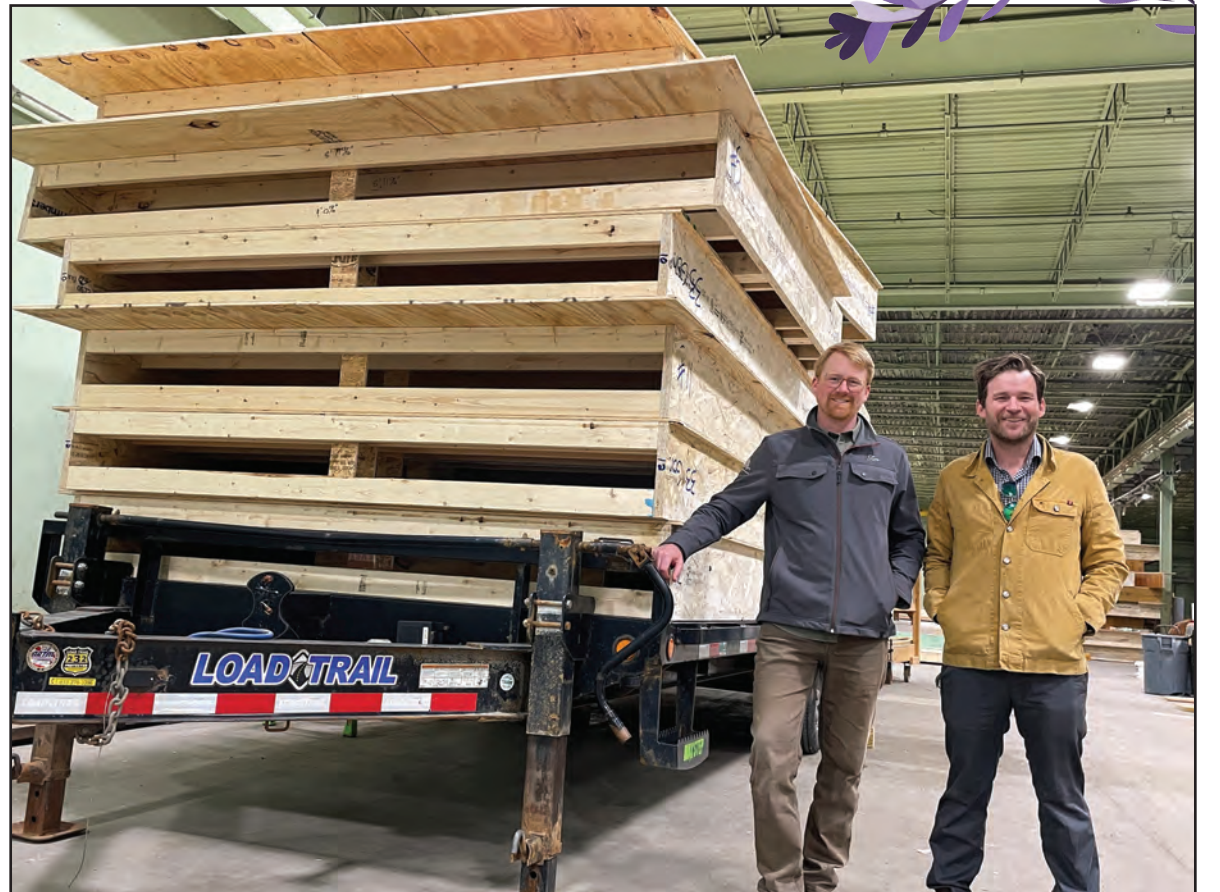
TIM STEELE, DIRECTOR of Silver Maple Construction's woodworks division (left), and Sean Flynn, the company's president, stand next to a stack of wall panels that will form the shell of a new Habitat for Humanity of Addison County home that's being built off Gorham Lane in Middlebury. Silver Maple's provision of the wall panels has been a huge assist to Habitat volunteers.
