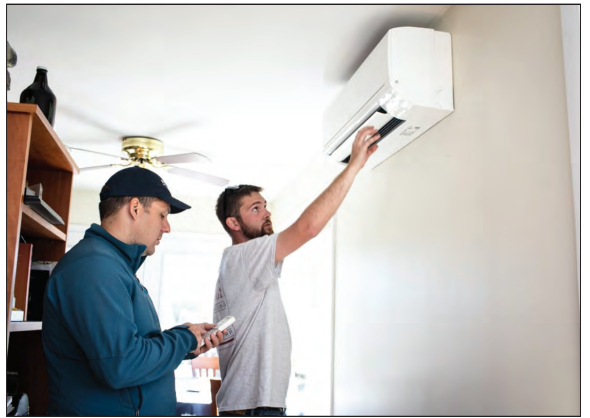
CODY STEPHENSON, A contractor with Vermont Energy, installs a heat pump in a Vermont home a few years back. Photo courtesy of Efficiency Vermont
