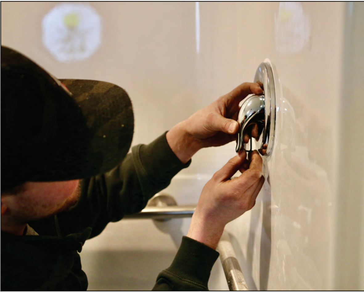
DUSTIN WHITCOMB OF Champlain Valley Plumbing and Heating uses an Allen wrench for the fiddly part of attaching a new shower tap in an East Middlebury home undergoing renovation.
