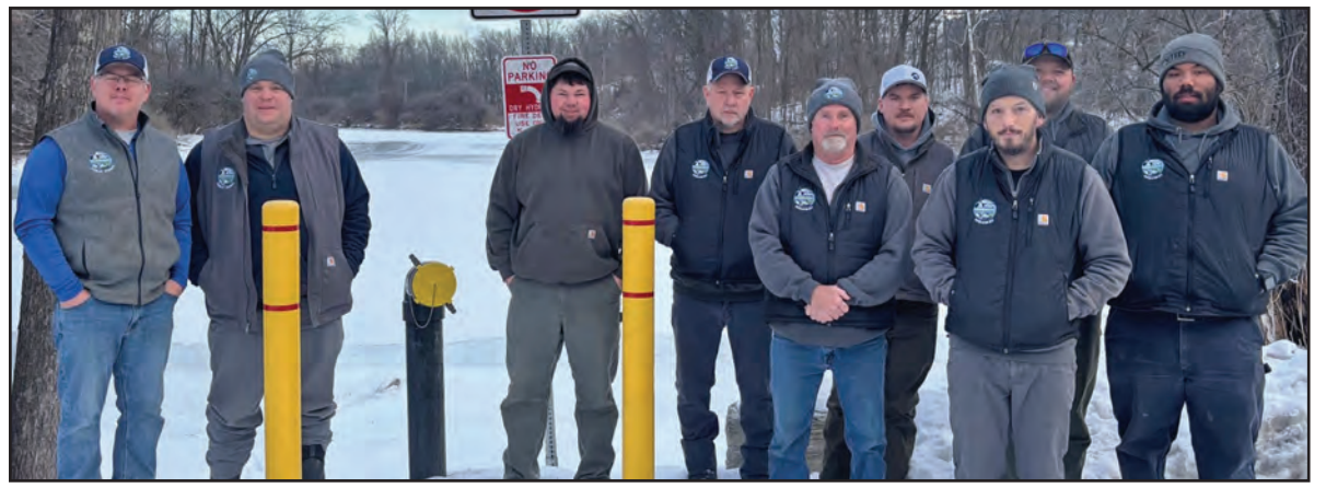
MEMBERS OF THE Middlebury Public Works Department check out the dry hydrant that was installed in the Frog Hollow section of Middlebury to give firefighters access to an abundant water supply in case of a blaze.
