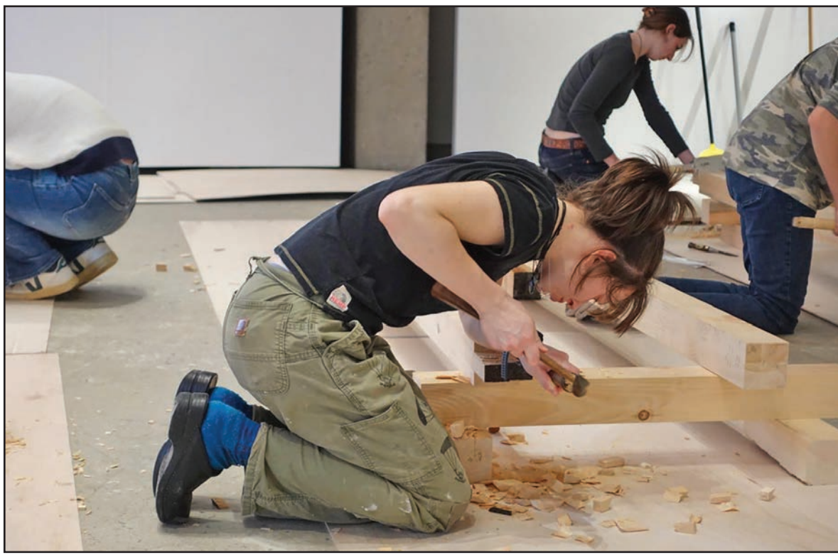
MIDDLEBURY COLLEGE STUDENTS work in silence to hone wooden pieces into the timber frame of a traditional Japanese tea house. This J-term class uses hands-on construction to explore the technical aspects of Japanese carpentry and to enlighten themselves on the cultural underpinnings of apprentice learning vs. Western styles of verbal learning.
