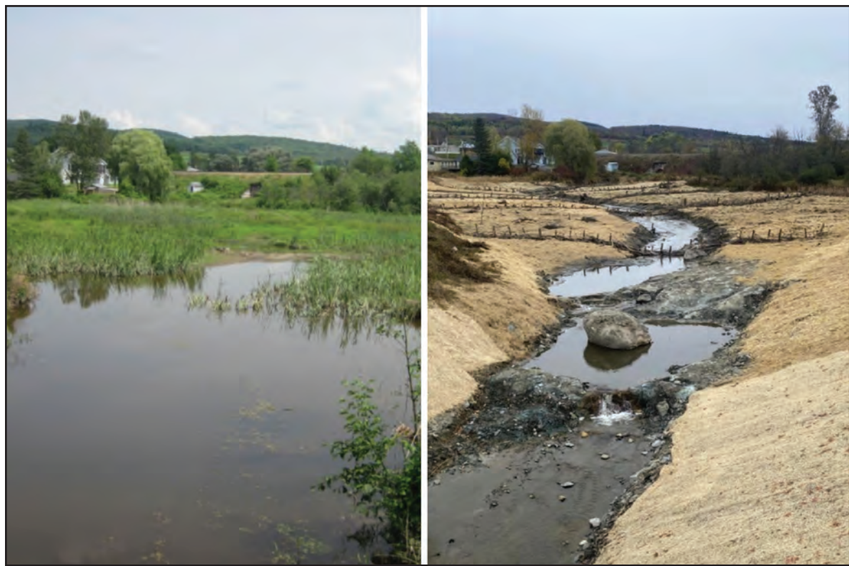
THIS SHOWS THE landscape before and soon after the removal of Newport's Sleeper Pond Dam in Oct. 2025.
