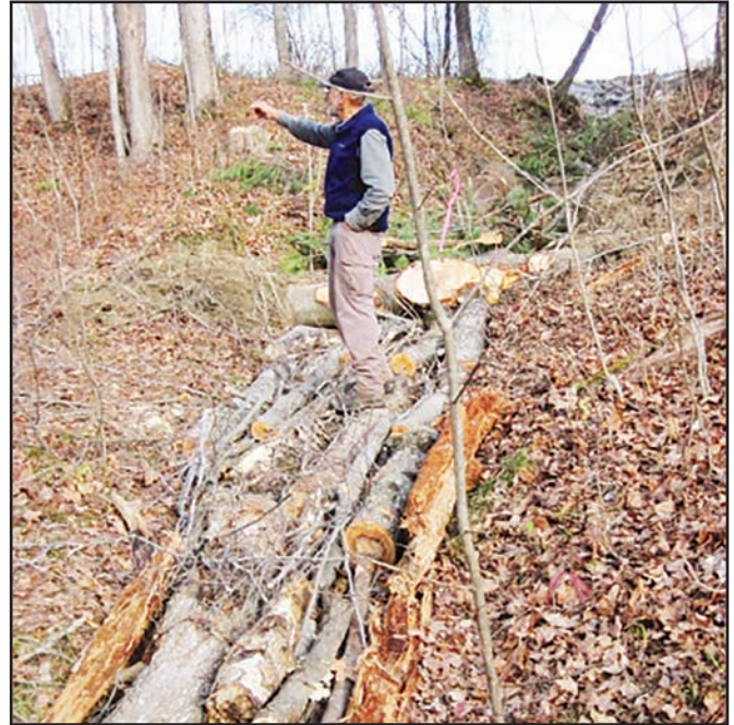
Engineers used trees and brush to fill gullies leading into Pond Brook as a “soft” method to stabilize the land and reduce erosion that was harming the water and the downstream watershed.
