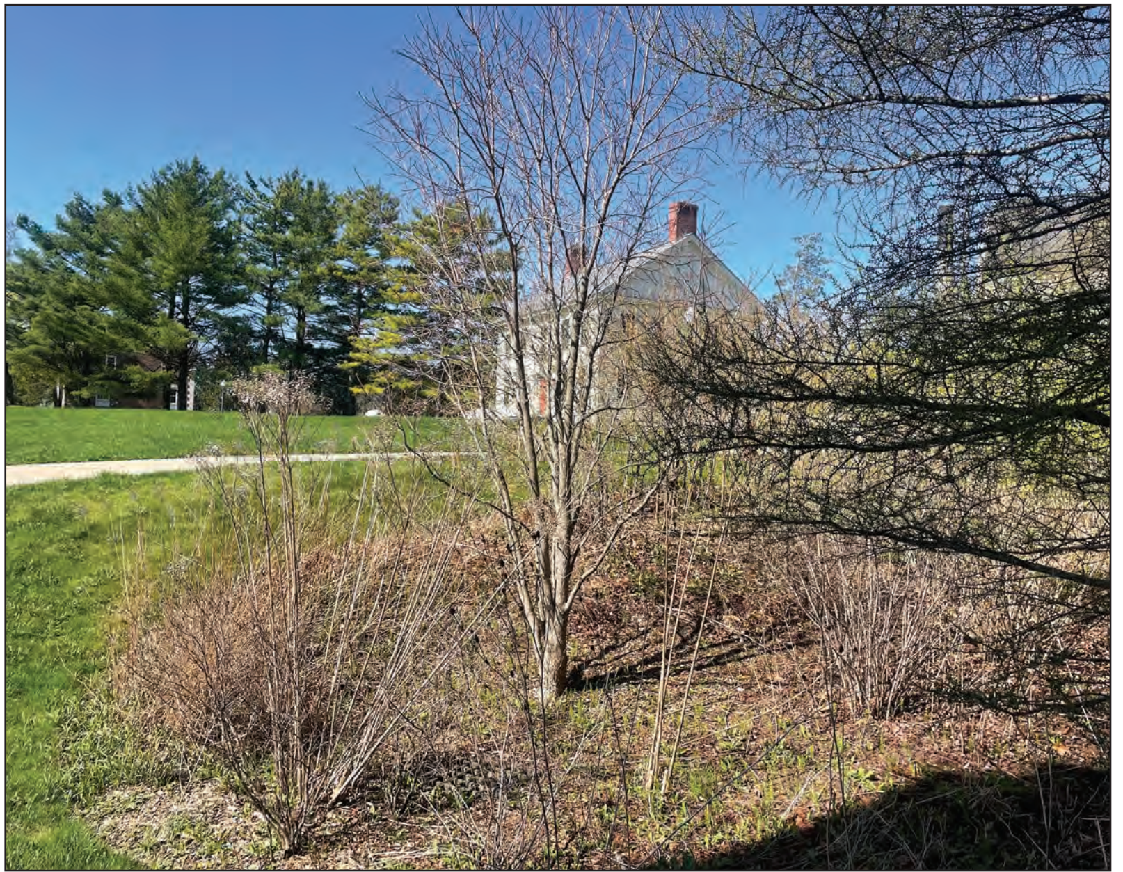
MIDDLEBURY COLLEGE TREATS stormwater on its campus through various types of green stormwater infrastructure, including stormwater retention and filtering features just outside the Axinn Center at Starr Library. A courtyard at the site has been graded and sloped to collect rainwater that flows off the roof into swales, which are broad, shallow channels that help convey and filter stormwater.
