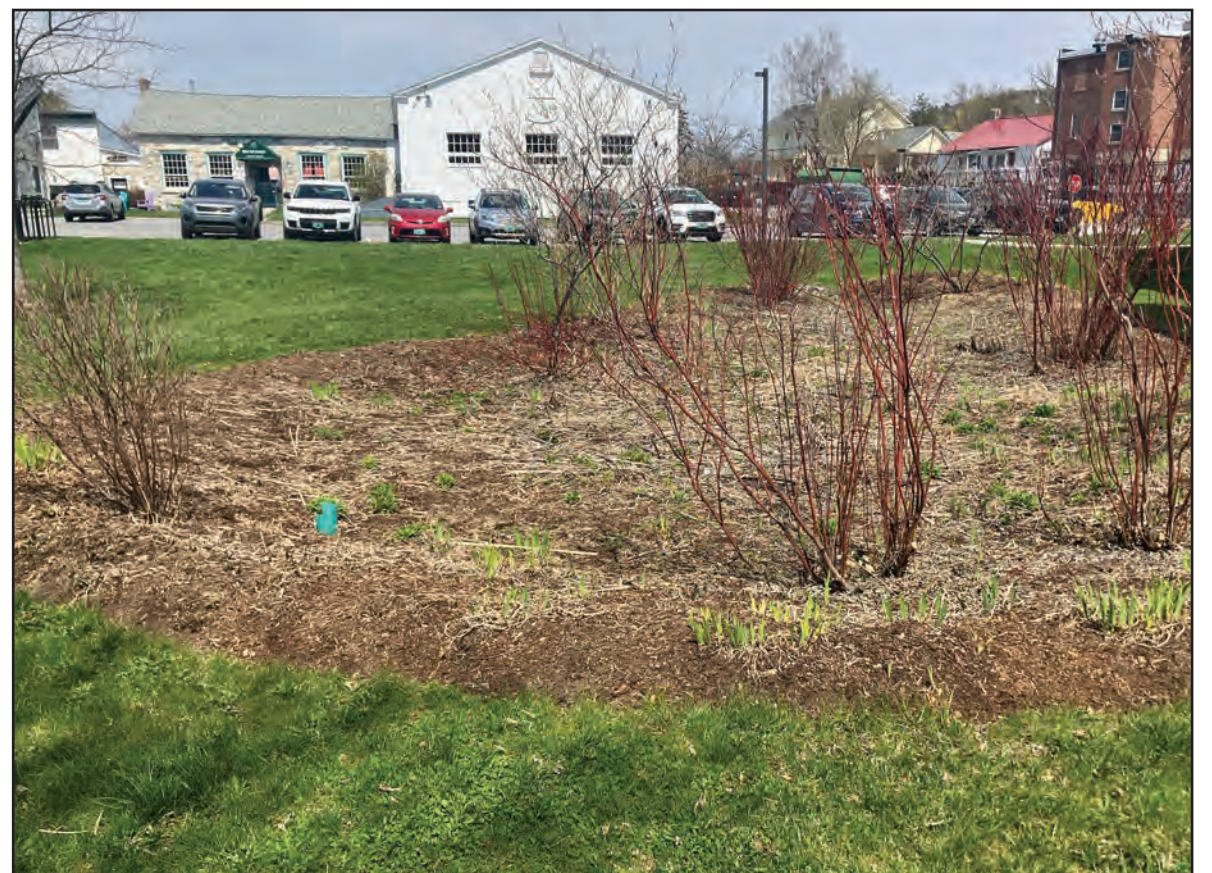
THIS RAIN GARDEN in Middlebury’s Marble Works complex is classically situated in a low-lying spot where it can collect and absorb rainwater and also filter some contaminants out of the water that runs off the nearby parking lot.
