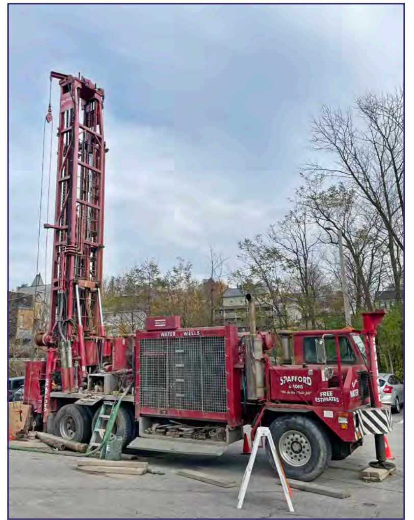
SIX TEST WELLS, including this one at the bottom of the ramp from the lower parking lot to the lot behind Ilsley Library, are being drilled to determine the potential for geothermal heating at the library and other downtown buildings.
