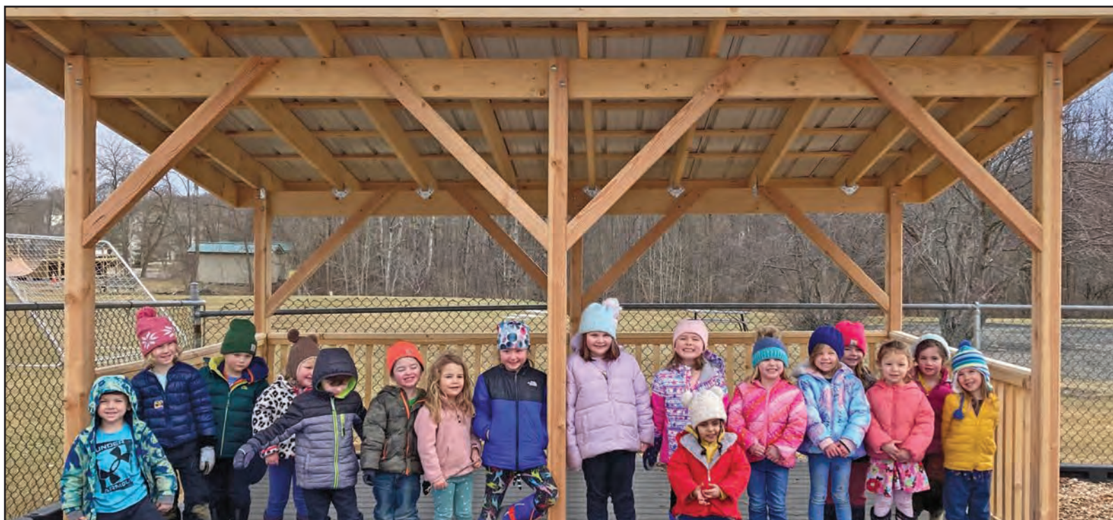
MARY HOGAN PRESCHOOLERS flush with excitement over their new lean-to and outdoor kitchen space, which students from the Hannaford Career Center constructed on the Mary Hogan playground.
