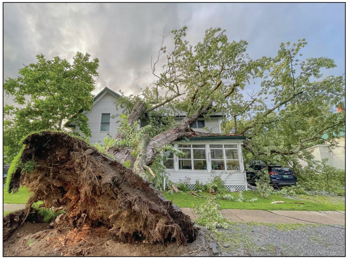
AS TROPICAL DEPRESSION Debby passed through Bristol on Friday, high winds knocked trees over on homes, including this one on Church Street. No injuries were reported.
