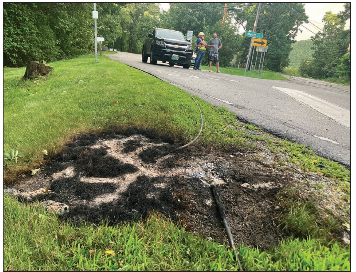
WHEN A TREE knocked over a utility pole off Case Street in Middlebury Friday evening, the broken electric line created a small fire on the ground near the entrance to Mead Lane. No one was hurt, but the road was closed for hours.
