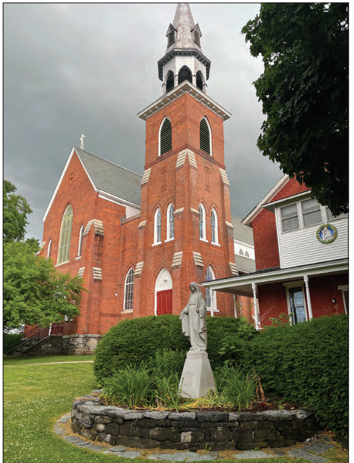
ST. PETER'S CATHOLIC Church on South Maple Street in Vergennes, which opened its doors in 1874, was built by parishioners volunteering their labor. Today's parishioners are embarking on ambitious effort they hope will prepare the church building for another 150 years.
