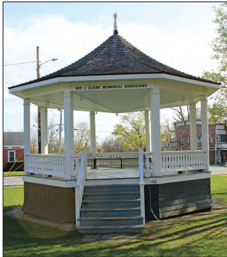
CHANGES ARE BEING proposed to the bandstand that has stood on the Bristol town green for 87 years. The selectboard said it would consider making it bigger and lower to the ground so it could accommodate more Bristol Band members without making them climb steps.
