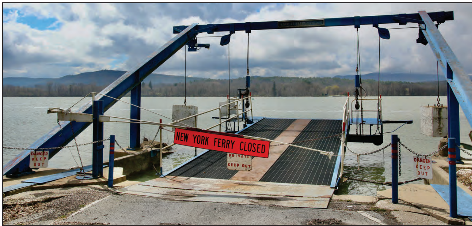
THE OWNER OF the historic Fort Ti Ferry said a planned May 1 service launch has been cast in doubt by an ongoing inspection and debris-recovery effort being staged by developers of the Champlain Hudson Power Express. That's a new cable sending electricity to New York City. Independent photo/Steve James
