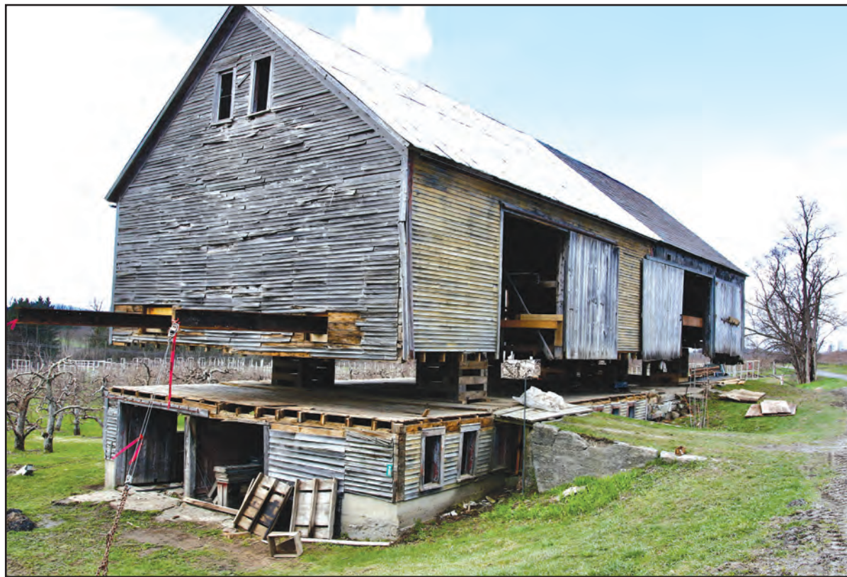
VERMONT HEAVY TIMBER has lifted the 40x80-foot bank barn facing Basin Harbor Road in Shoreham as the first stage of a $200,000 restoration project. The renovated first floor will provide an open space where Douglas Orchards plans to seasonally offer community gatherings and storage during winter. Independent photo/Steve James
