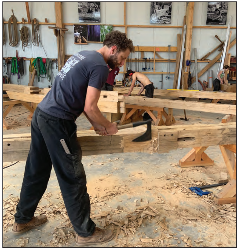
LINCOLN CARPENTER WILL Wallace-Gusakov uses a broadaxe to hand-hew an oak beam for the Notre Dame cathedral's nave roof frame. The same technique would have been used by the medieval carpenters who constructed the original frame nearly 800 years ago.
