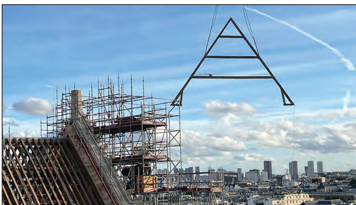
A WOODEN TRUSS constructed by Lincoln’s Will Wallace-Gusakov and other carpenters is flown on to the Notre-Dame de Paris cathedral. Wallace-Gusakov and a team of woodworkers last year rebuilt several trusses for the cathedral’s nave roof frame, which was destroyed by a fire in 2019. Photo courtesy of Will Wallace-Gusakov
