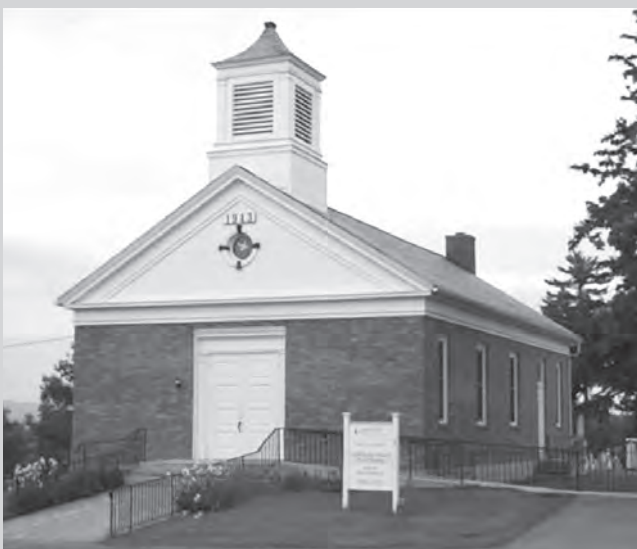
The Bridport Church • CCCC 54/72 Middle Road • Bridport, VT
