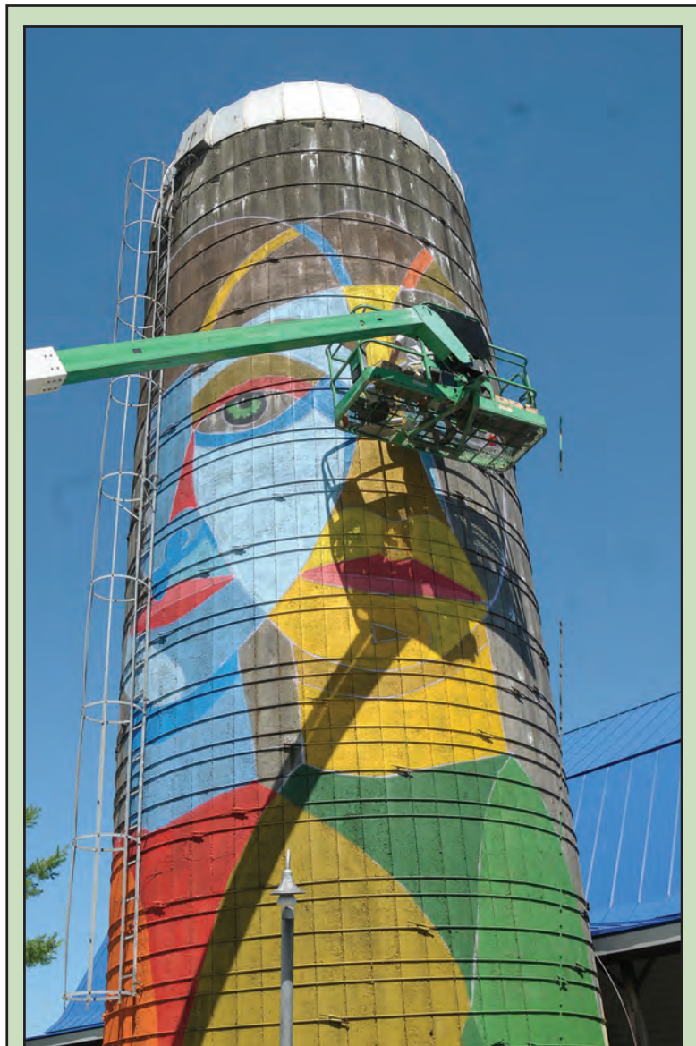
CHRIS MURRAY GOT a lift to enable him, and Olivia Lane, to paint a mural on the silo at Middlebury's Bridge School in July 2018. This week the deteriorating silo was dismantled for safety reasons.
